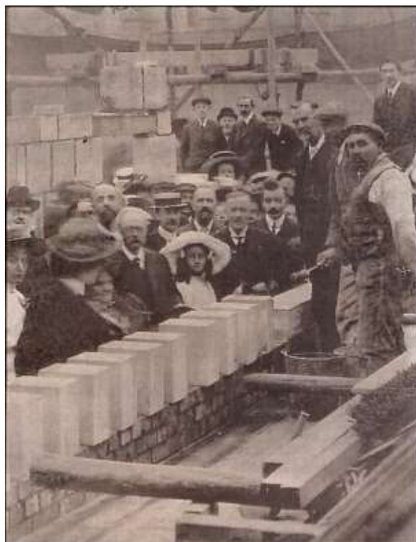
Laying the foundation stone for the Institute, c.1910.
